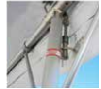
Tensioning Hook to valance
