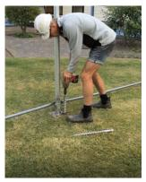
Pre drill pilot hole with impact wrench (this determines holding power). Earth Anchor can then be installed. NB Pilot drill should be as close to anchor length as possible.
