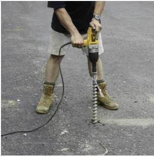
Pre drill pilot hole with impact wrench (this determines holding power). Earth Anchor can then be installed.
